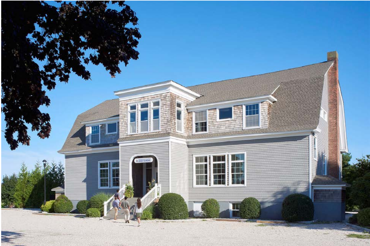
Riverhead Charter High School; renovated in 2022.
